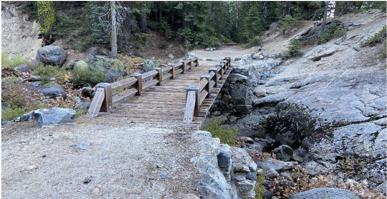
Cascade Creek Bridge
